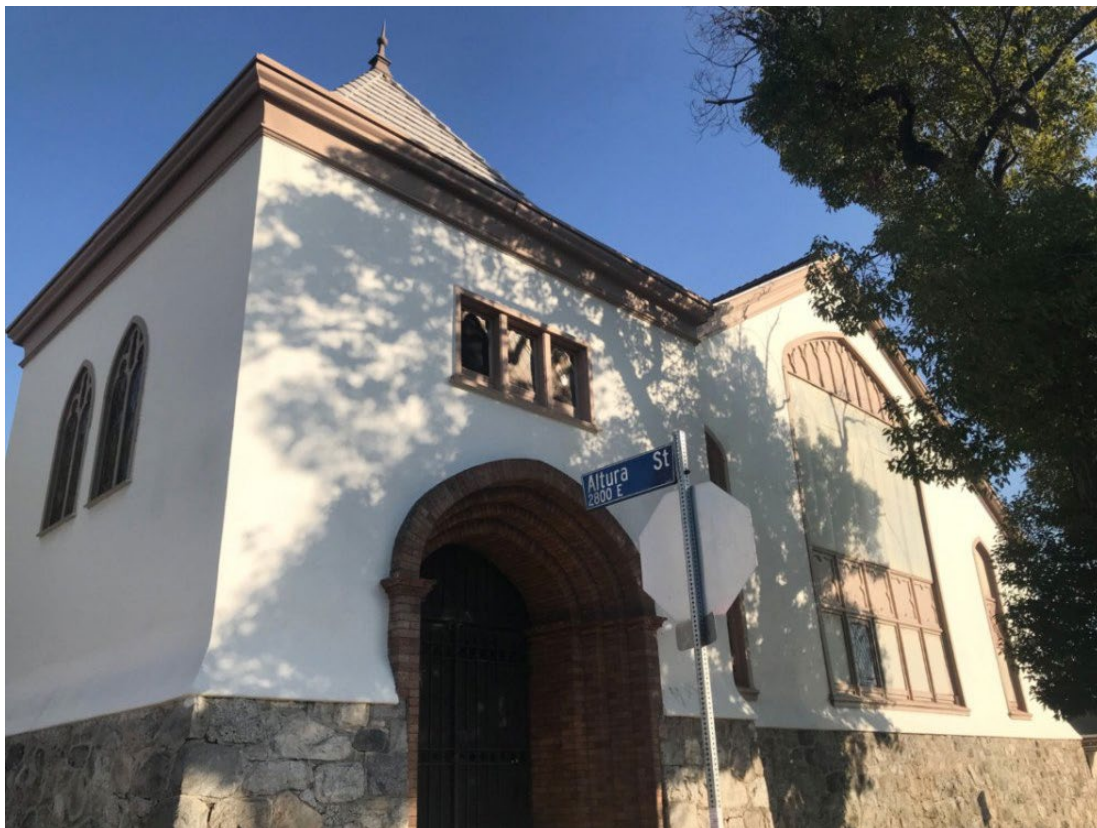
The Church of the Epiphany, in the Lincoln Heights neighbourhood of Los Angeles, recently earned a spot on the National Register of Historic Places. The church is known as the birthplace of the Chicano movement in the 1960s. Photographed on Thursday, 4TH February, 2021. PICTURE: RNS/Alejandra Molina
